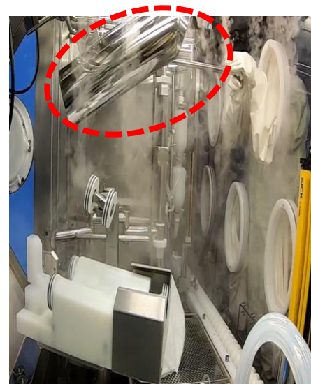
[Installation of chute]
